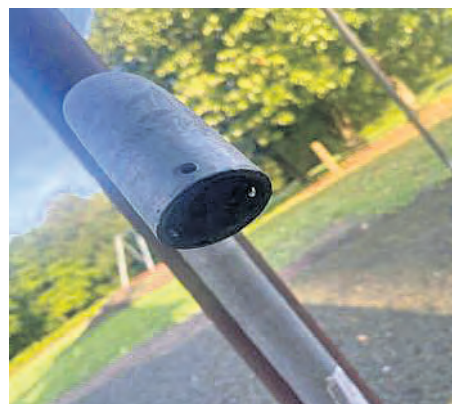
Sharp edges around the talk tubes where caps have not been fitted, which could cause risk of cuts.
